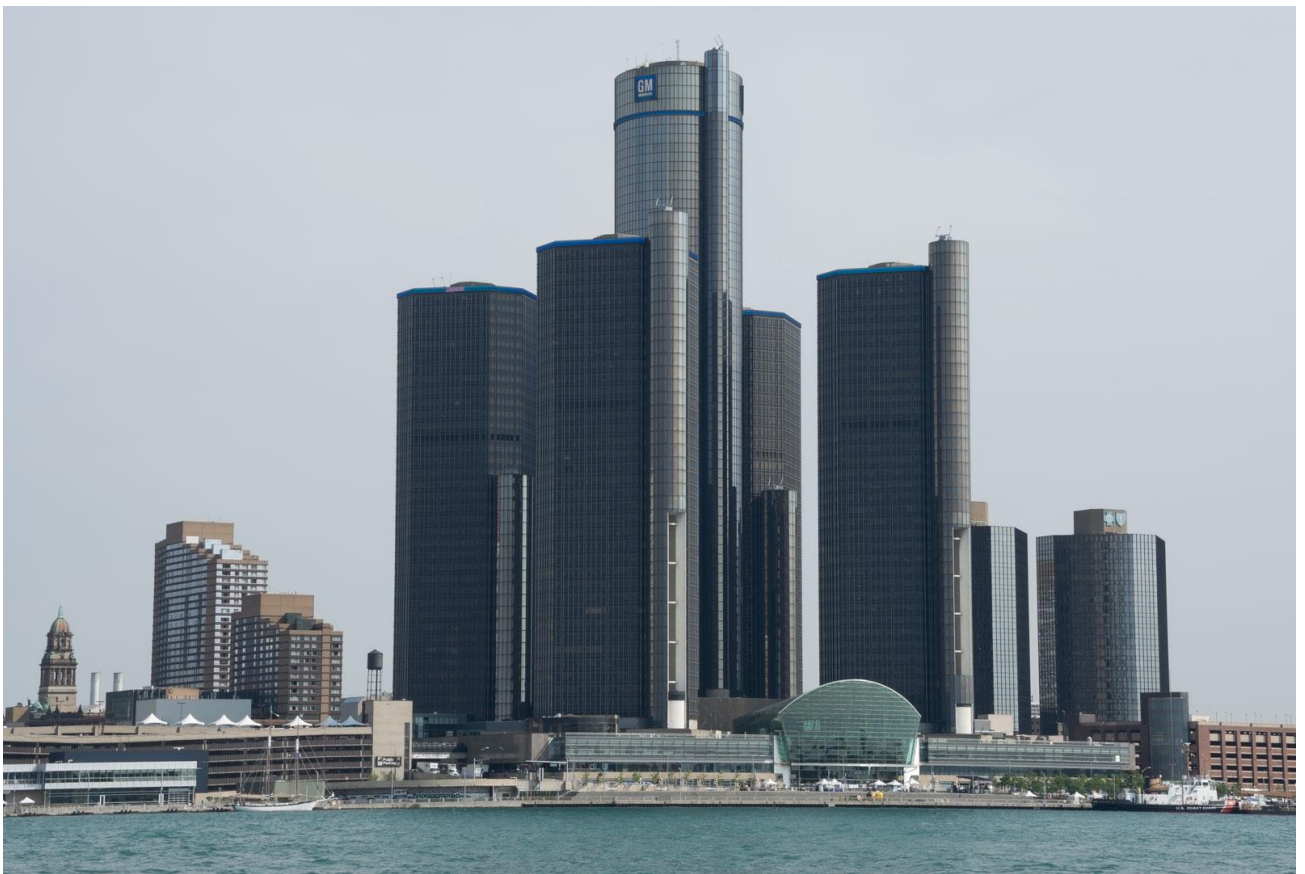
Picture. 4. Headquarter of General Motors
